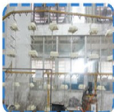
Painting production lines on the 1st Floor
